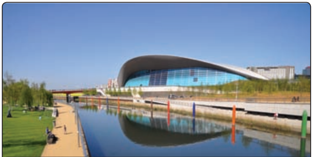
Aquatics Centre of the Queen Elizabeth Olympic Park in Stratford, East London
